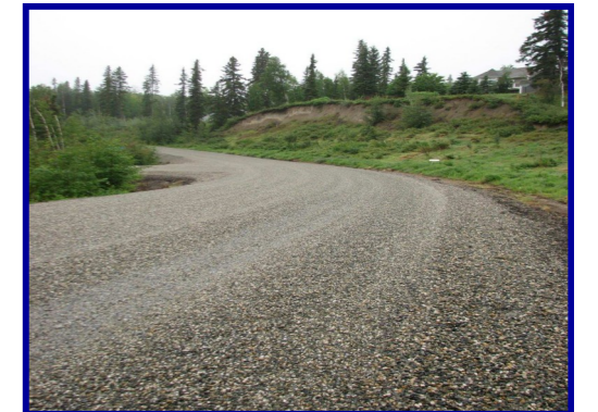
Chip sealing of Old Chena Ridge Road
