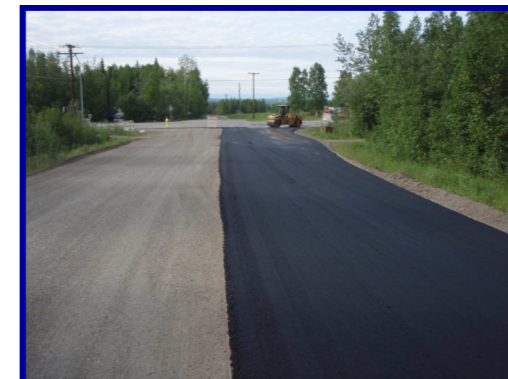
Asphalt paving of Summit Drive
